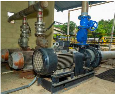
Water Treatment Efficiency Pumps Replacement Project
