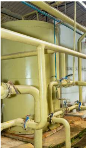
Sand Filter Replacement
